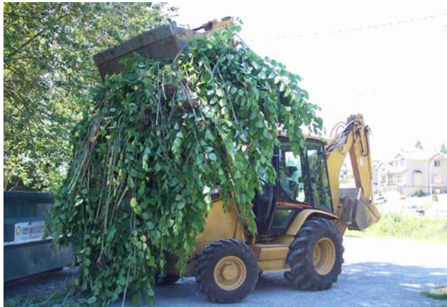
Heavy equipment at work
